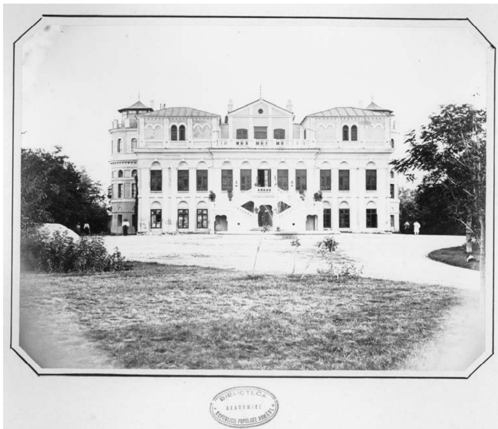
Fig. 29. Franz Duschek, The Oteteleşanu Palace at Măgurele – the main entrance, albumen print from a wet collodion negative, Library of the Romanian Academy.
